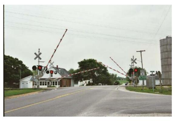
Cantilevered Flashing Light Signals and Gates -- Ash Street in Springfield
